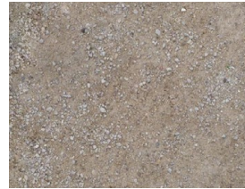
Img 22 - Self binding gravel (Source: LUC)
