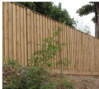
Img 28 - Timber acoustic fencing (Source: thewildegroupp.co.uk)
